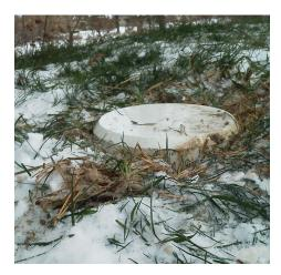
The caps on the mound need to be removed in order to inspect the lateral lines inside the mound. These access caps need to be of a screw in and out design with easy screw top removal. This will enable the technician to remove the caps easily without damaging the piping in the mound. If possible, the technician will by using the discharge pump, flush the mound lateral lines to help clear the lines.
