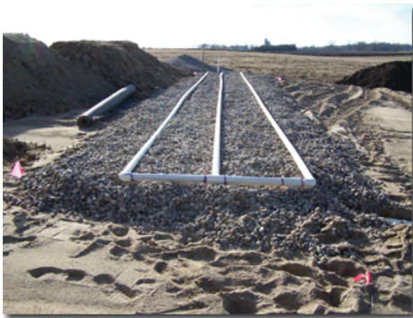
Mound septic system in process
